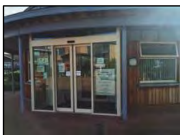
Denham Medical Centre, Denham Garden Village
